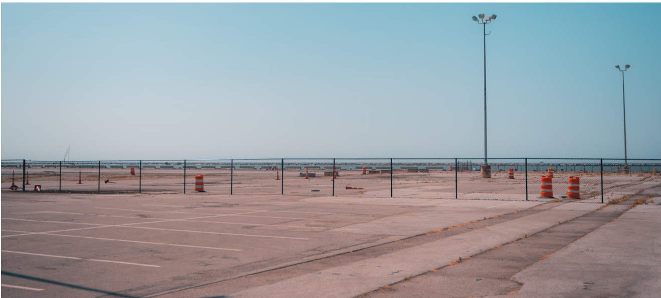
An asphalt lot without a single tree. Such a surface heats far more than a shaded one during the day and admits practically no water: the whole volume of rainfall reaches the storm sewer within minutes, forming the very peak the sewer must then be sized for.
